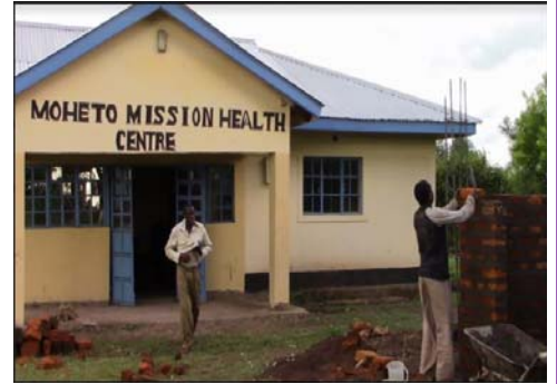
The center now has refrigeration.
